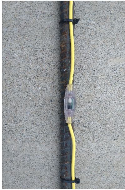
Thermal Sensor Cable attached to rebar
